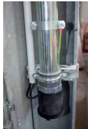
Antistatic vacuum inlet with ground connection
